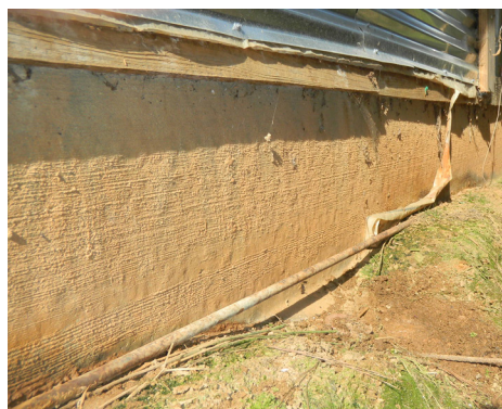
Figure 8. Examples of foundations undermined by erosion.
