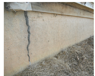
Figure 11. Foundation cracking due to rotation/settling.
