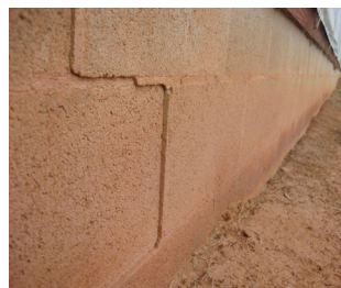
Figure 11. Foundation cracking due to rotation/settling.
