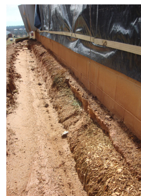
Figure 5. An exposed foundation due to erosion.
