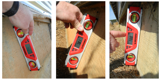
Figure 12. Measuring the angle of rotation of a concrete stem wall.
