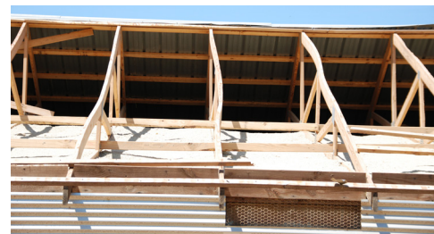
Figure 25. Bracing of trusses is essential to keep trusses vertical and to help carry loads along the length of the house.
