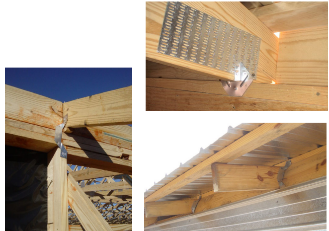
Figure 24. Trusses tied to the top of a wall using "hurricane straps."
