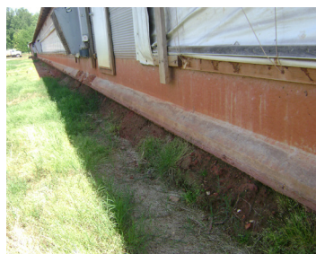
Figure 5. An exposed foundation due to erosion.
