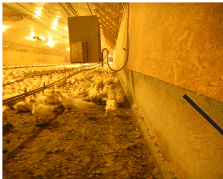
Figure 10. Interior Erosion: Soil should be added to maintain structural integrity.
