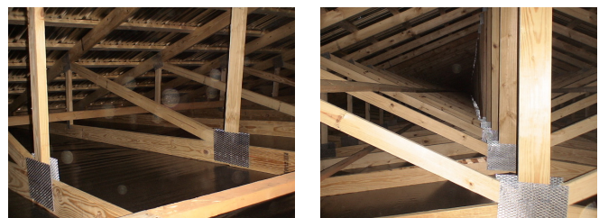
Figure 24. Trusses tied to the top of a wall using "hurricane straps."
