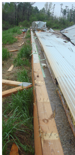
Figure 17. Nails loaded in withdrawal allowing pullout.
